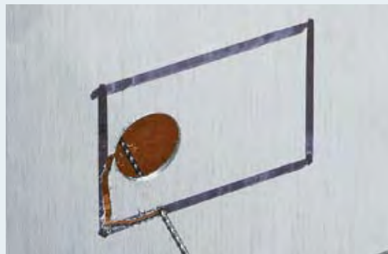
◀ Odd Shapes. A starter hole is all you need to cut an opening with a spiral blade.
